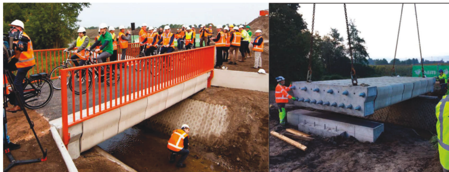
FIGURE 30: Installation process and overall structure of concrete 3D printing bridge [60].
