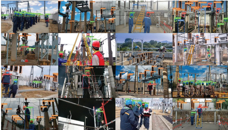
FIGURE 5: The detection performance of the FFA-YOLOv7 model. The operators wearing safety helmets and safety belts are highlighted with green bounding boxes. Those who are not wearing safety helmets, not wearing safety belts, or violating safety regulations are marked with red bounding boxes. The insulators and ladders are, respectively, indicated by orange and blue bounding boxes.
