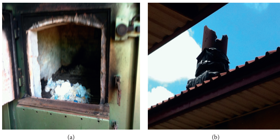
FIGURE 11: Imported incinerator at Brong Regional Hospital, Sunyani. (a) Combustion chamber. (b) Chimney without APCD.
