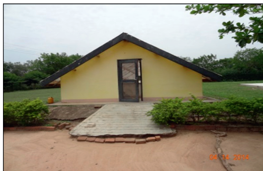
FIGURE 1: Pictorial representation of the concrete solar dryer (CSD).
