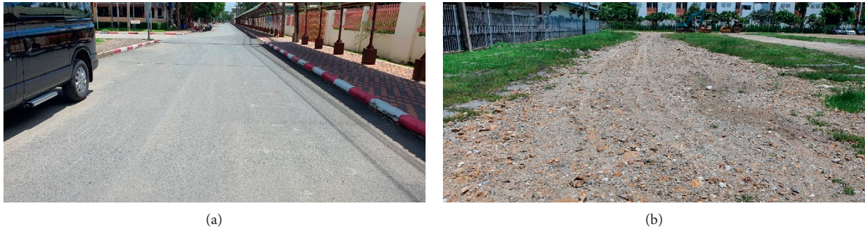
FIGURE 10: Road surface conditions used in case studies. (a) Smooth road (cement road type). (b) Rough road (gravel road type).
