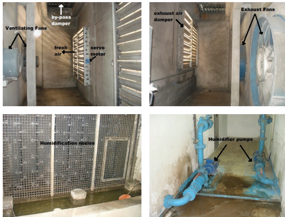
FIGURE 2: General view of humidification and air supplier units of controlled system.
