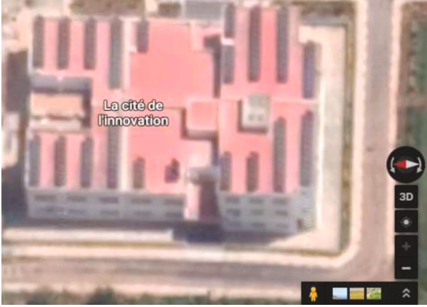
FIGURE 1: A view of the building taken by Google Maps.
