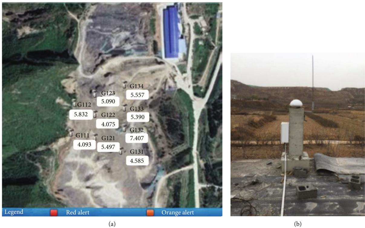
FIGURE 8: The layout of the monitoring points and installed GNSS monitoring equipment.
