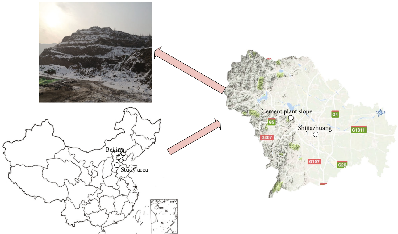
FIGURE 7: The location and actual view of the slope studied.
