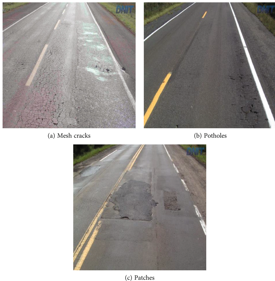
FIGURE 8: Pavement defects.
