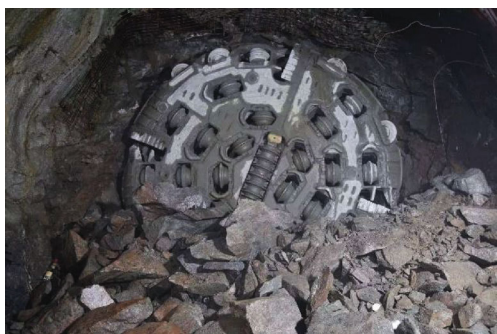
FIGURE 2: Rock breaking by TBM cutter head.
