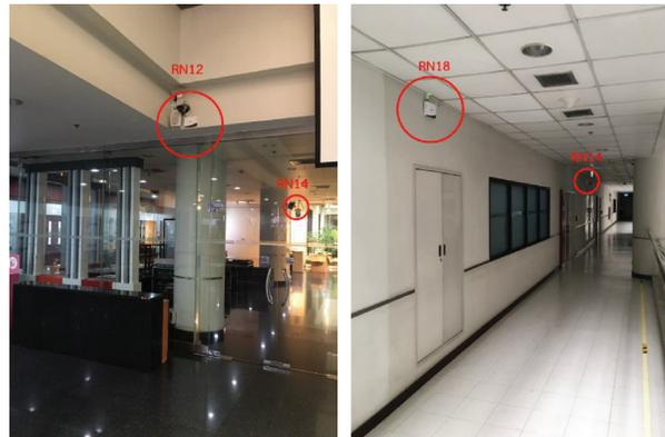
FIGURE 15: Examples of installed RNs inside the NETEC building. (a) RNs for the 1<sup>st</sup> floor area. (b) RNs for the 3<sup>rd</sup> floor area.
