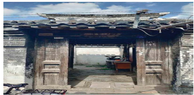
FIGURE 4: Well-preserved old building.
