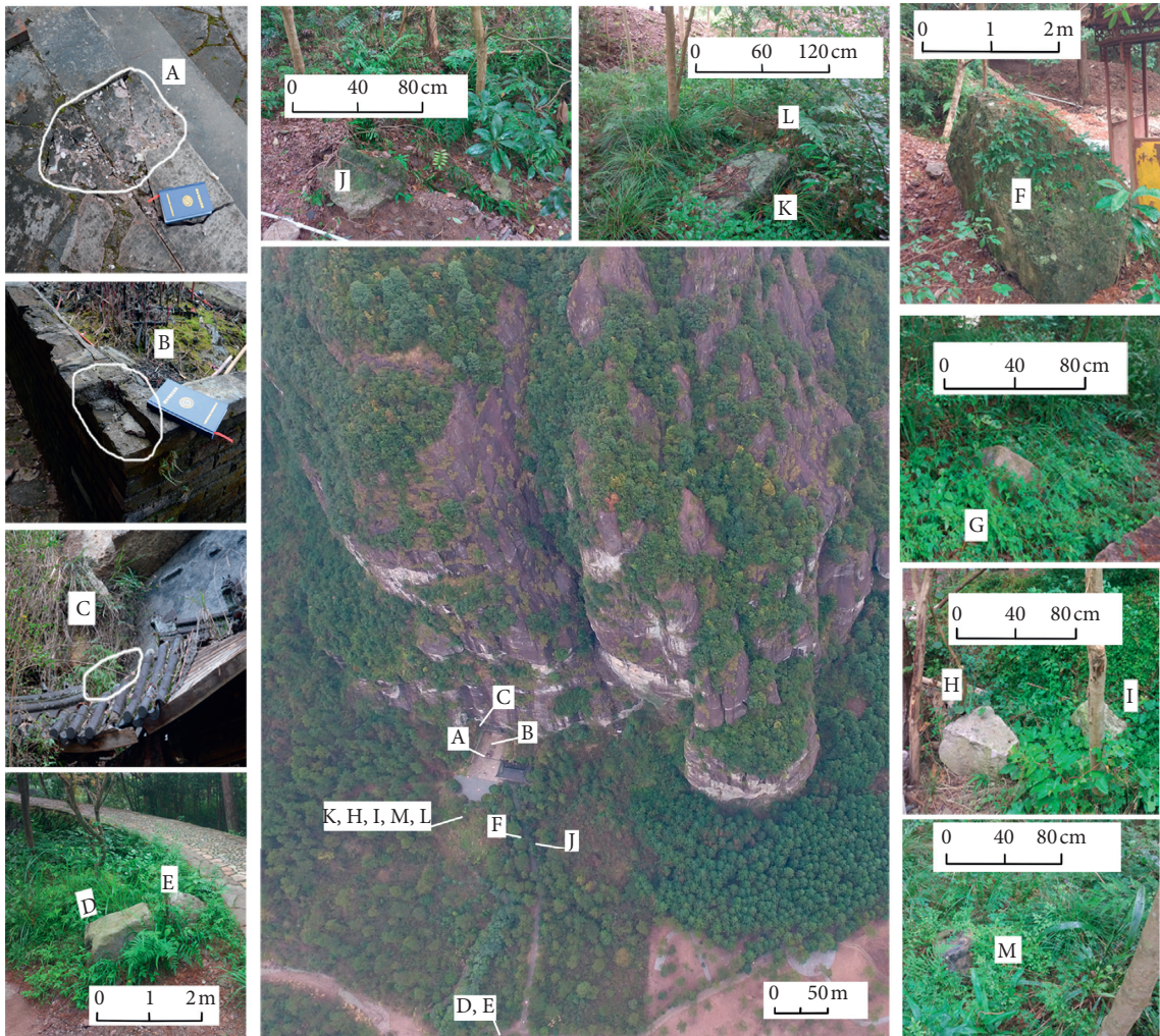
FIGURE 5: Historical rockfall survey results for the Guanyindong Slope.
