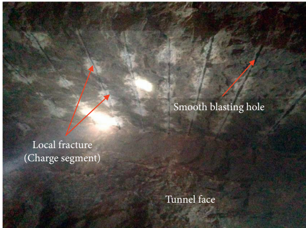
FIGURE 10: Macroscopic characteristics of surrounding rock along the borehole after the on-site smooth blasting.
