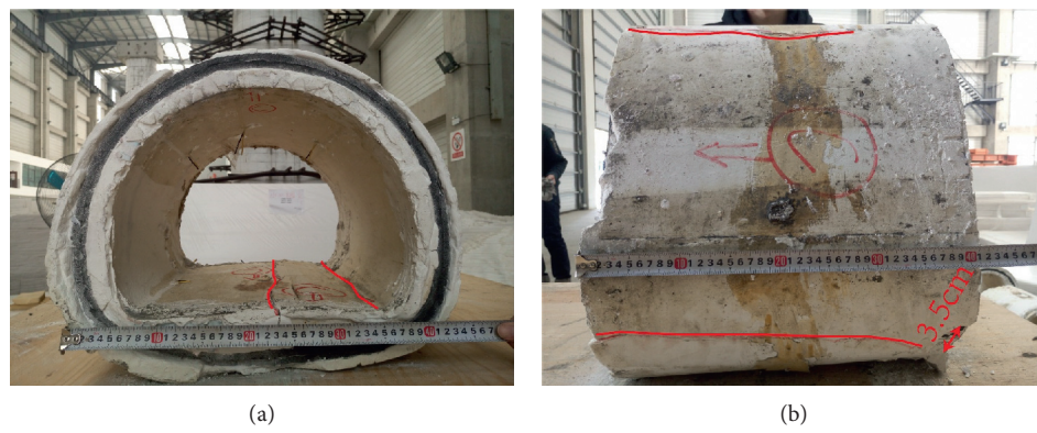
FIGURE 17: Damage of composite lining with 2 cm buffer layer. (a) Transversal surface. (b) Longitudinal surface.
