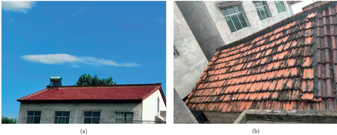
FIGURE 1: (a) Roof of a new building. (b) A roof covered with dust and moss.
