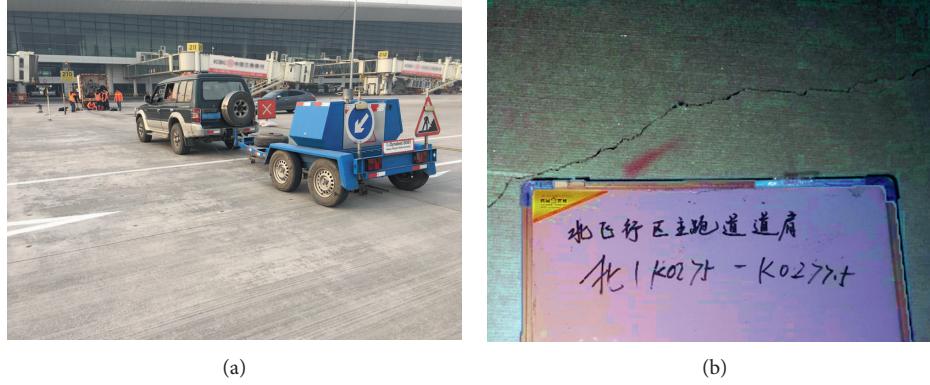
FIGURE 1: Field inspection of airport runway: (a) inspection equipment; (b) crack detection.
