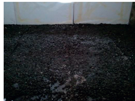
FIGURE 7: Gravel cemented at box bottom.
