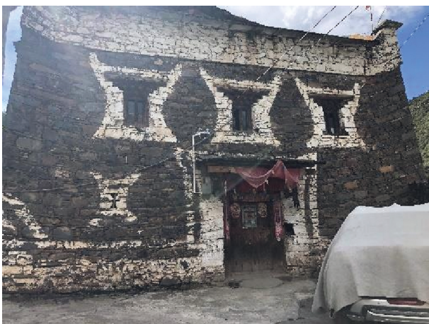
FIGURE 5: The arc formed by the retraction of the wall and the improvement of the corner brings a sense of stability.
