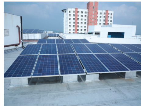
FIGURE 3: Arrangement of Rooftop solar panels of VIT University, Chennai.
