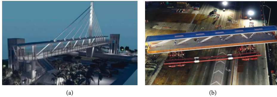
FIGURE 6: The actual scene diagram and collapsed scenario of the American FIU bridge. (a) A rendering of the FIU human bridge. (b) The FIU bridge construction collapse site.
