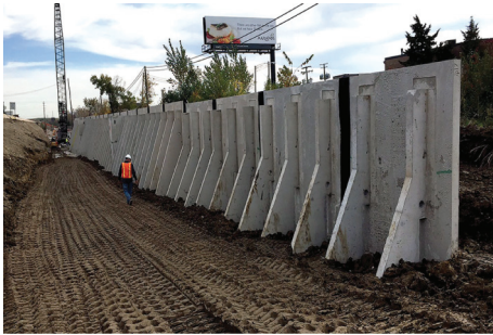
FIGURE 3: Precast retaining wall.
