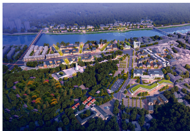
FIGURE 24: A partial aerial view of the planning and design of Red Army Square.
