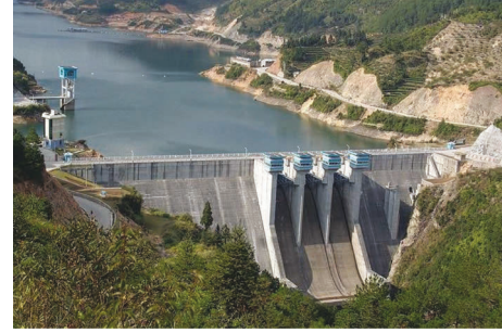
FIGURE 3: Photo of the gravity dam.
