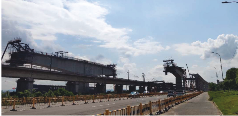
FIGURE 6: Bridge site on construction.
