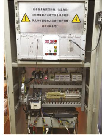
FIGURE 17: Sinusoidal constant current dimmer.
