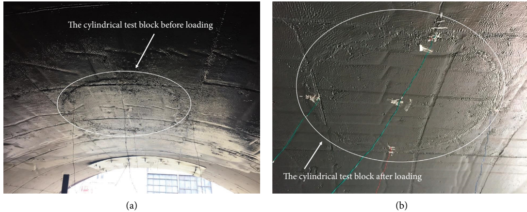
FIGURE 31: The appearance of the spray film material of the tunnel arch cylinder test block. (a) Before loading. (b) After loading.
