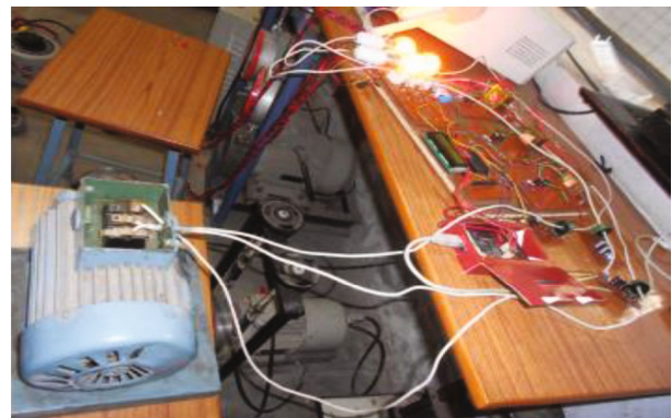
FIGURE 9: Three-phase induction motor running with protection system.
