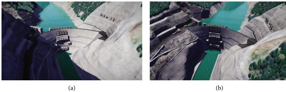
FIGURE 10: The solar radiation effects on the summer solstice. (a) At 9:00 am. (b) At 12:00 am.
