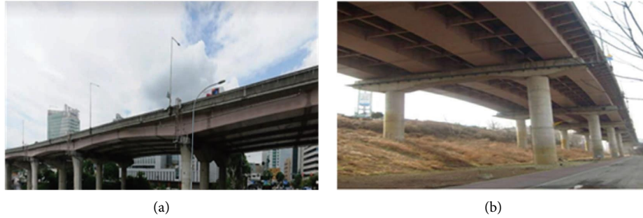
FIGURE 4: Test bed: overpass bridge.
