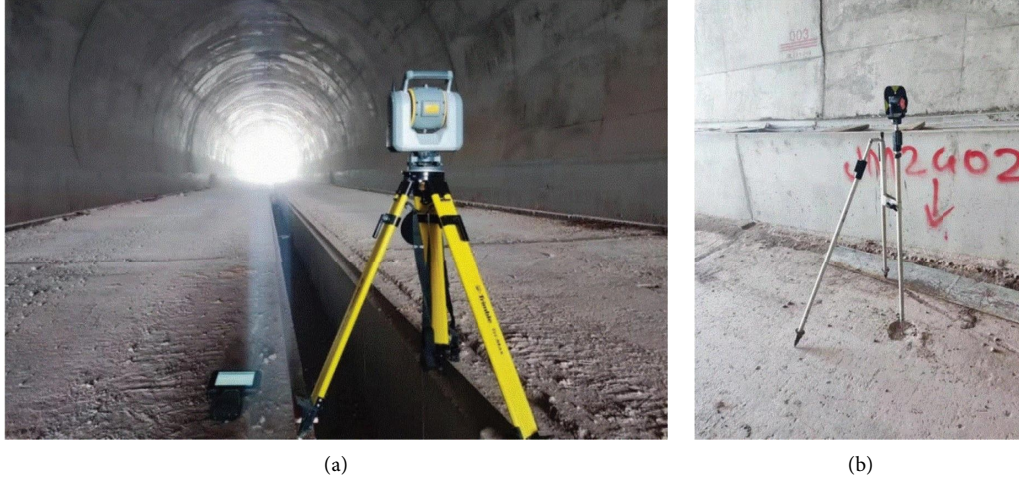
FIGURE 2: Schematic diagram of data acquisition. (a) Laser scanner placement schematic. (b) Prismatic and railway tunnel control points.
