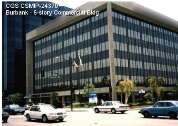
FIGURE 6: Exterior elevation of Burbank building.
