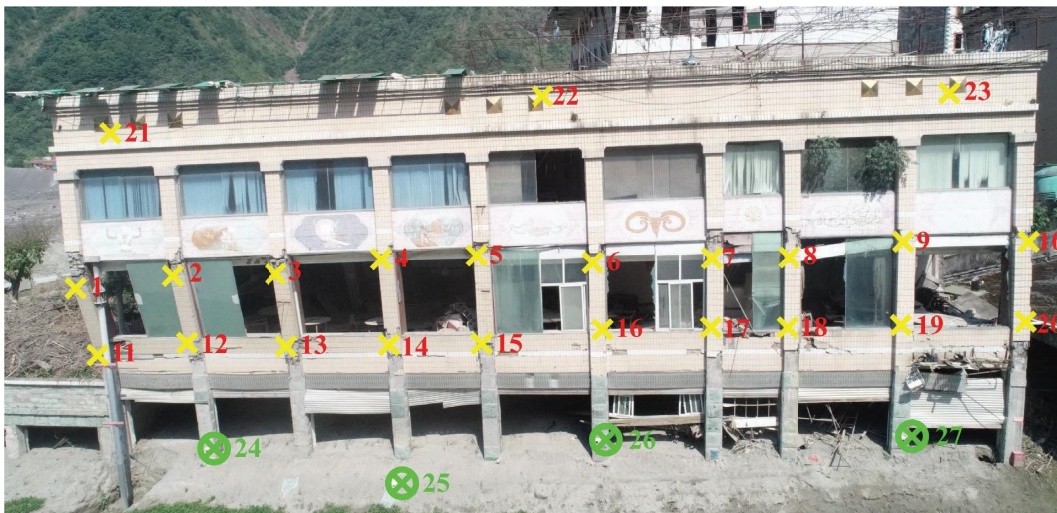
FIGURE 10: Overview of the three-story frame structure and layout of GCPs.
