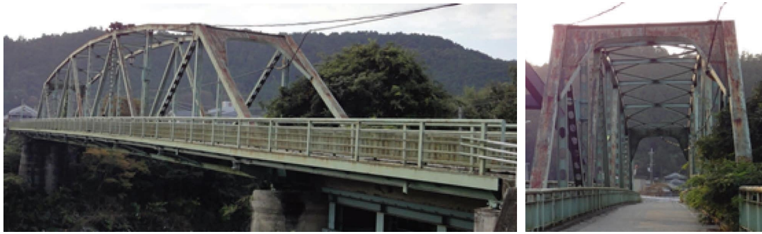
FIGURE 2: Photographs of the target bridge [41].
