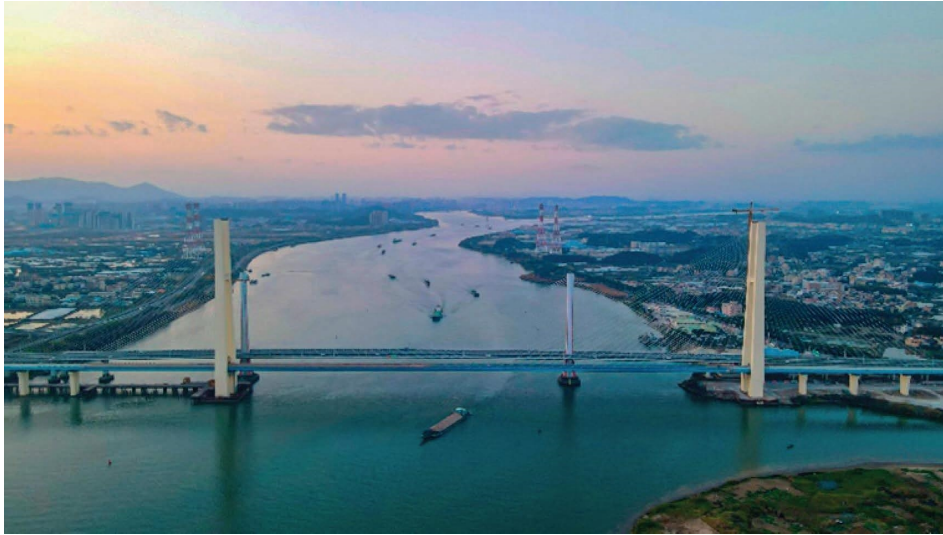
FIGURE 8: Aerial photograph of the experiment bridge.
