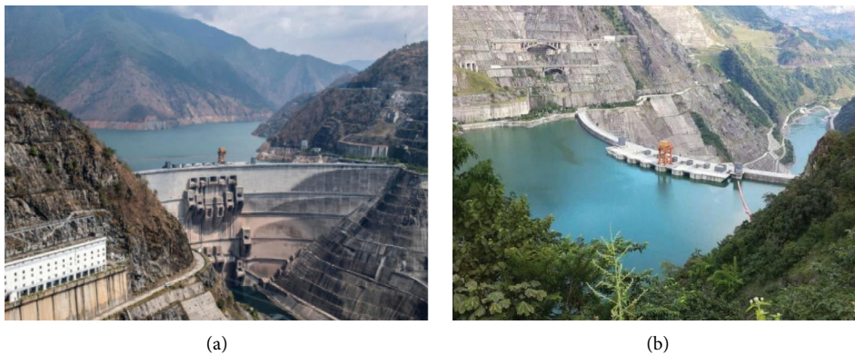
FIGURE 4: Aerial view of the dam: (a) downstream view and (b) upstream view.
