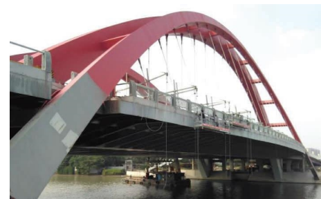
FIGURE 8: The investigated bridge.
