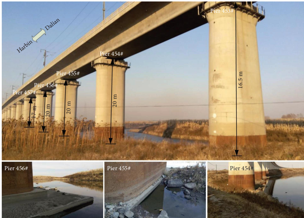
FIGURE 11: Schematic of pier 453#~457# in the 2 nd Songhua River bridge.
