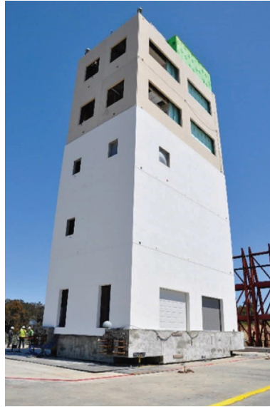
FIGURE 12: Full-scale building in the BNCS project.
