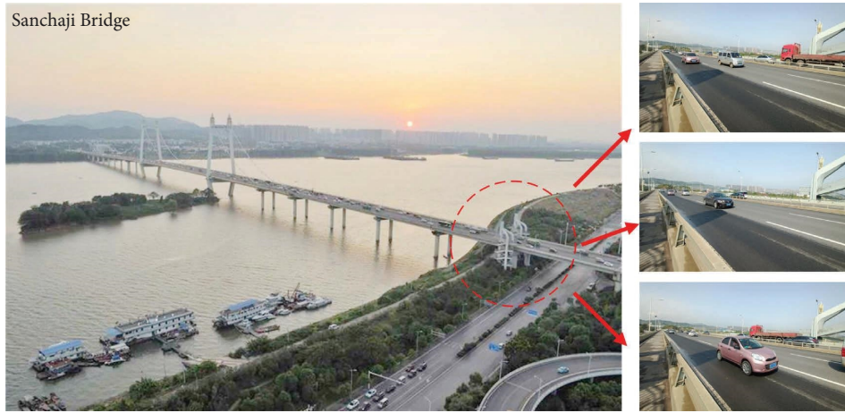
FIGURE 12: The location of the camera on the Sanchaji highway bridge over the Xiangjiang River in Changsha, China.
