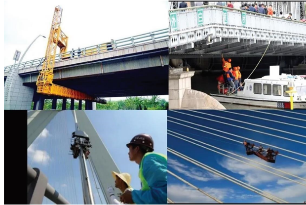
FIGURE 1: Common artificial bridge inspection methods.
