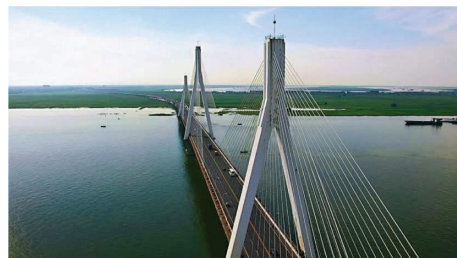
FIGURE 8: The steel truss girder suspension bridge in this study.
