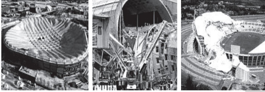
FIGURE 1: Collapse accident diagram of the stadium.
