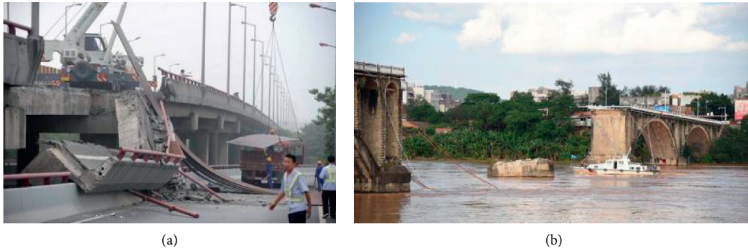
FIGURE 1: Bridge collapse accident.
