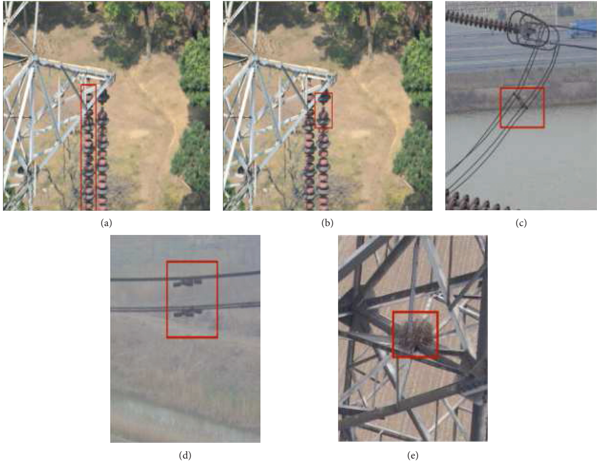
FIGURE 8: Detection target: (a) insulator, (b) insulator defect, (c) spacer, (d) shock hammer, and (e) bird nest.
