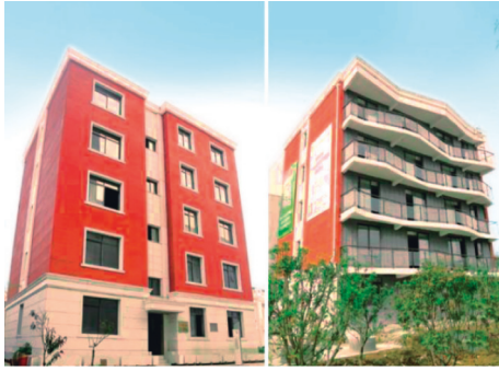
FIGURE 3: The world's tallest 3D printed building.
