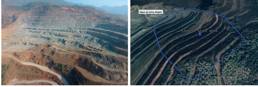
FIGURE 1: Status of Dahongshan open pit mine slope.
