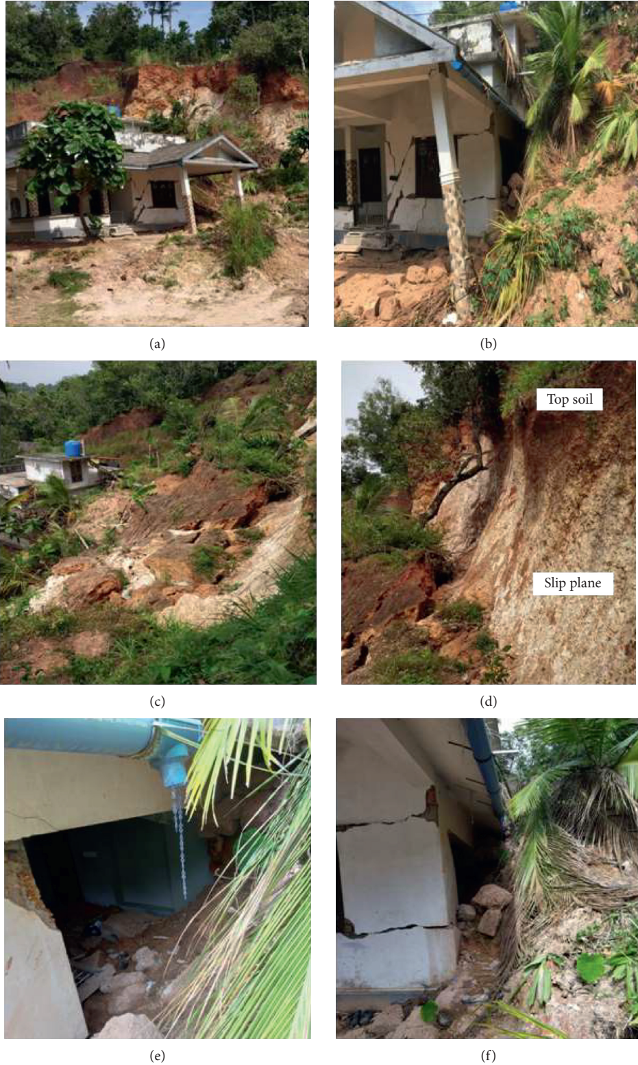
FIGURE 2: View of building failure. (a) View of the damaged house with vertical cut. (b) Elevation of damaged building. (c) Sliding part of the failed cut. (d) View of vertical cut failure. (e) Detailed view of the damaged portion. (f) Outside view of the damaged portion.
