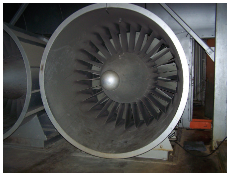
FIGURE 2: Axial vane fan located at the 10 x 10 SWT.
