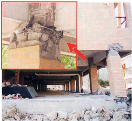
FIGURE 2: Damage of the bottom columns of a 6-story building [9].
