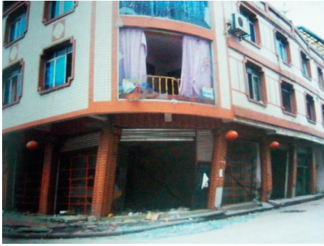
FIGURE 1: Damage of a 3-story frame structure [8].
