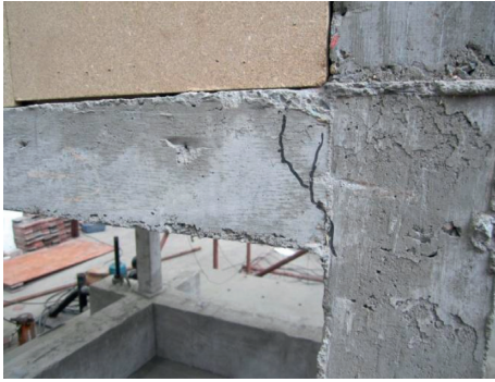
FIGURE 11: Diagonal cracks in a beam of straw frame.
