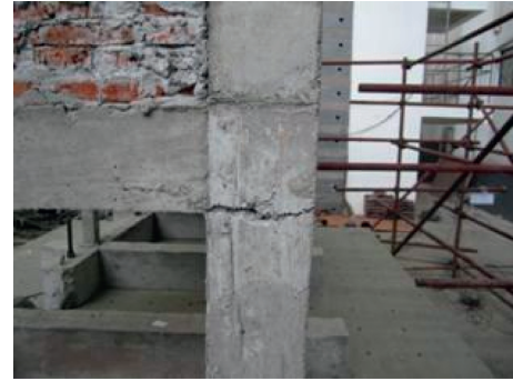
FIGURE 12: Crack in the bottom column of brick frame.
