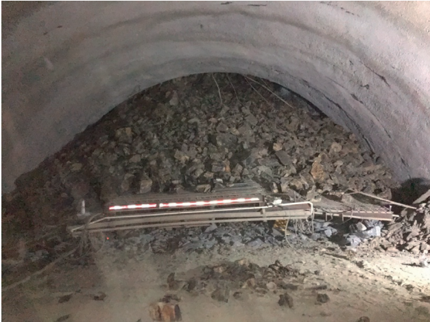
FIGURE 1: Collapse of the roof induced by a karst cave located above a highway tunnel.
